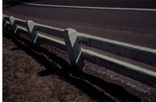
Columbia River Highway guardrail with steel-backing to meet federal crash tests requirements
