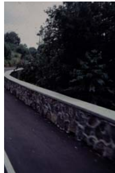
Concrete reinforced, stone-faced barrier wall, Kona, Hawaii
