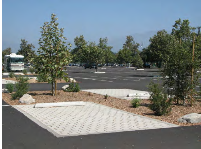
Permeable paving installed in Rose Bowl parking lot for the Brookside Park BMP Project (CDM, 2007)
