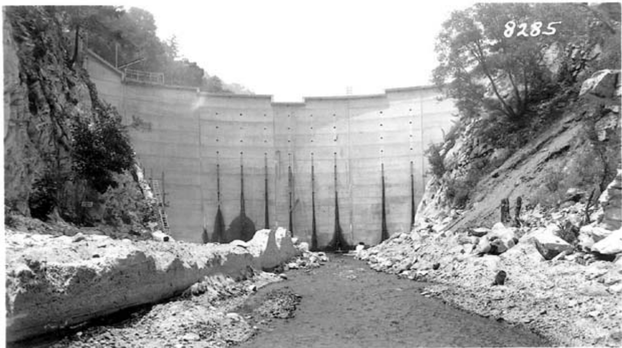
Scour downstream of Brown Mountain Dam shortly after construction June, 1943
