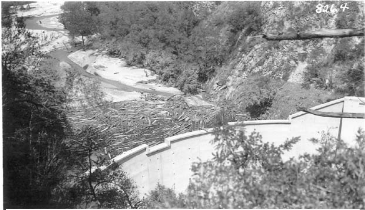
Debris and sediment accumulation above Brown Mountain Dam shortly after completion, March 1943
