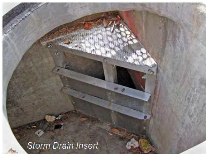
Storm Drain Insert Trash capture device installed in Rose Bowl parking lot for the Brookside Park BMP Project (CDM, 2007)
