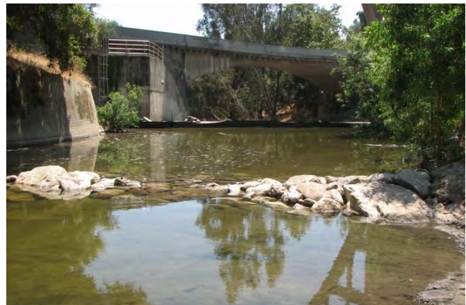
Downstream weir constructed in Central Arroyo Seco for Brookside Park BMP Project (CDM, 2007)
