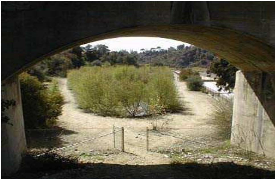
Access to the Lower Arroyo under the Colorado Bridge
