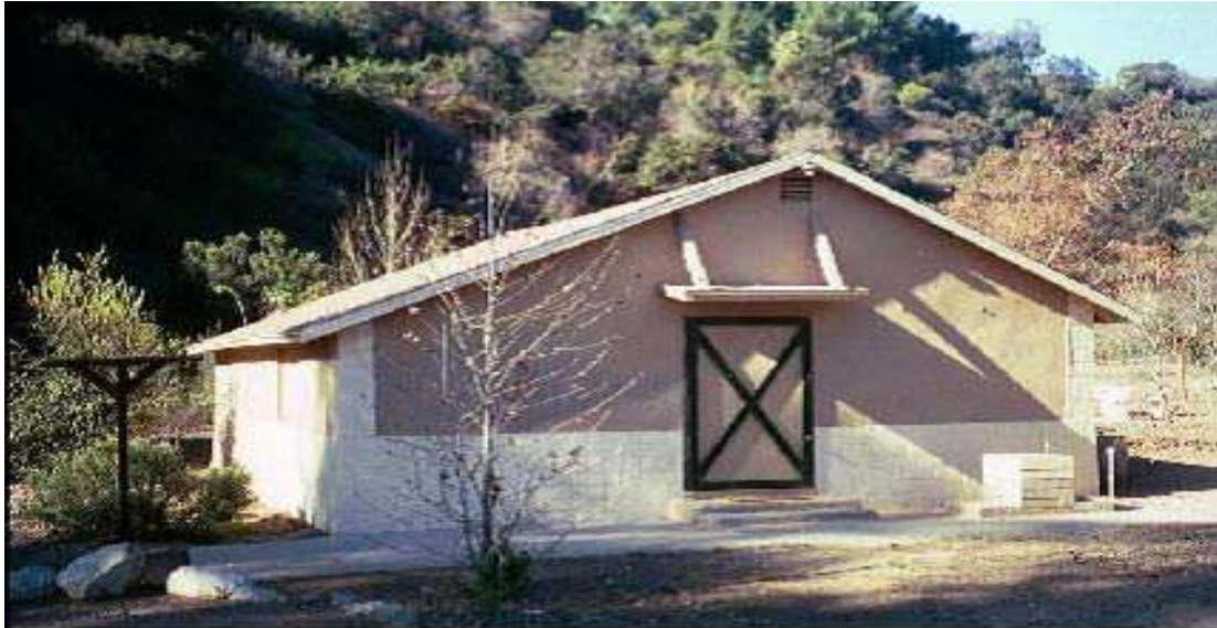
The Archer's Clubhouse before it was damaged by fire
