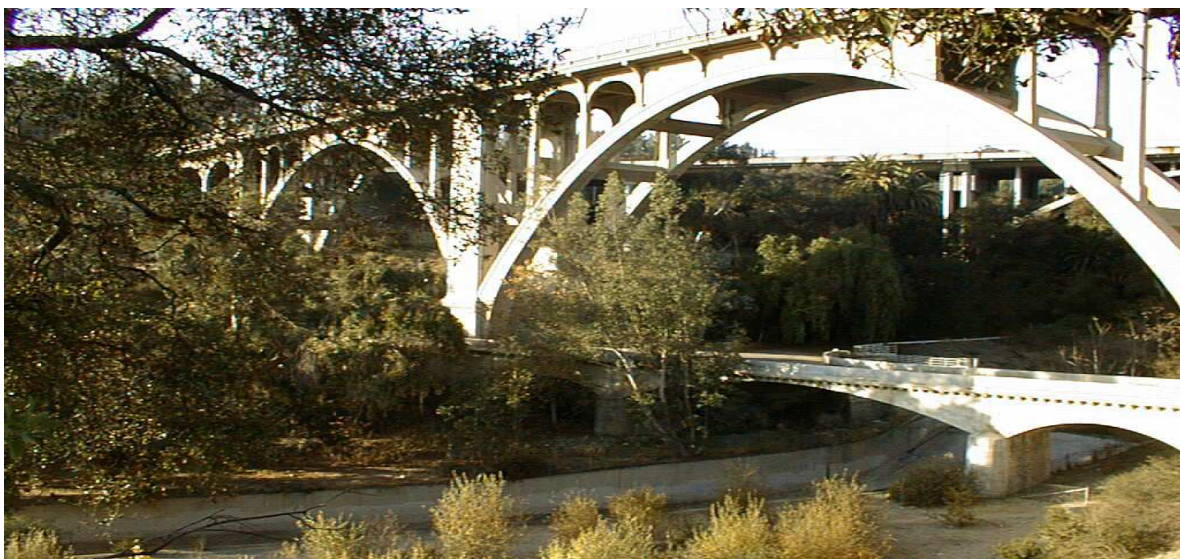
Parker-Mayberry Bridge below the Colorado St. Bridge
