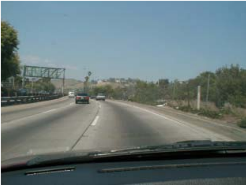
A motorist's view of the Parkway
