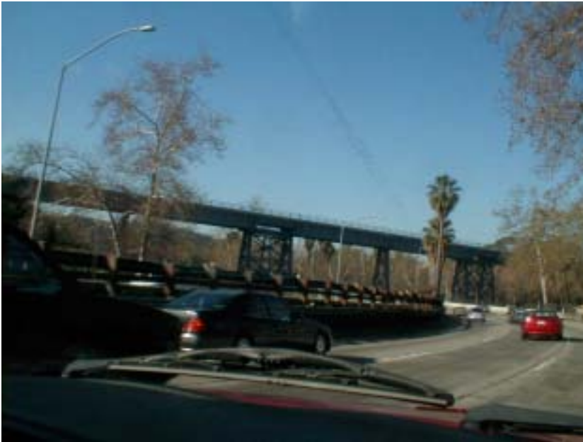
Santa Fe Railroad Bridge
