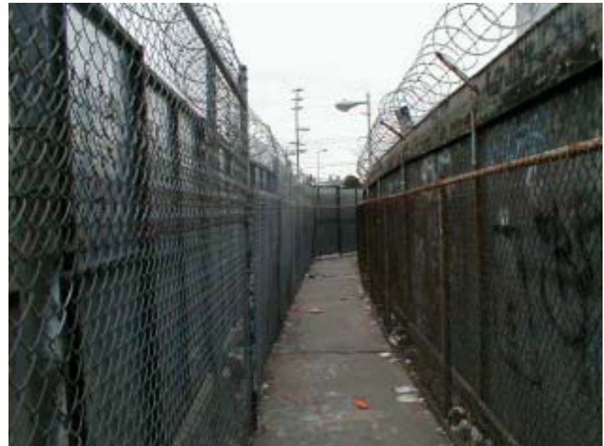
Cypress Street Pedestrian Overpass
