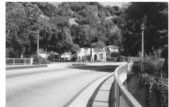
Avenue 52 Bridge and green spaces
