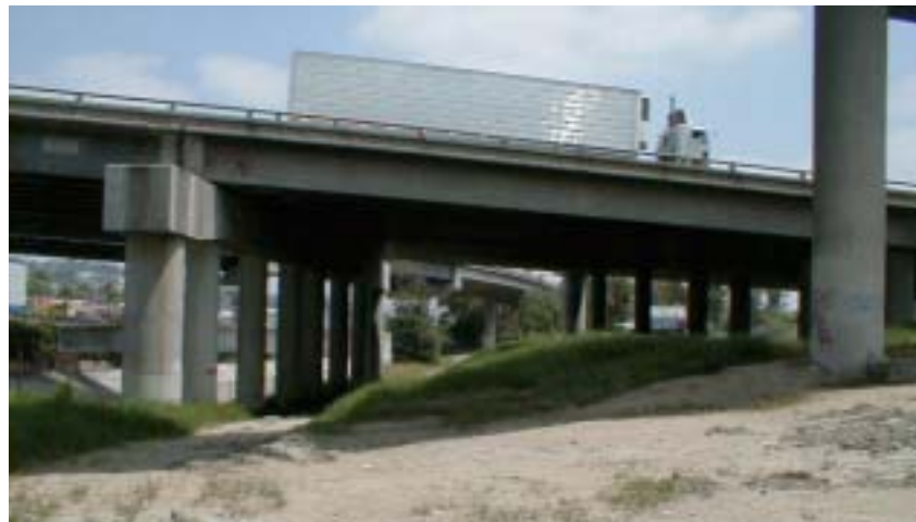
View under Interstate 5 overpass
