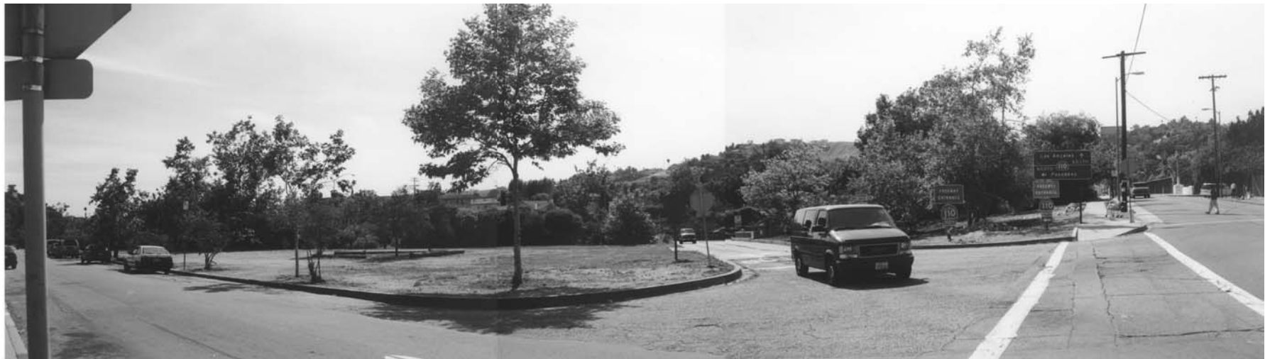
Avenue 43 offramp intersection: current conditions
