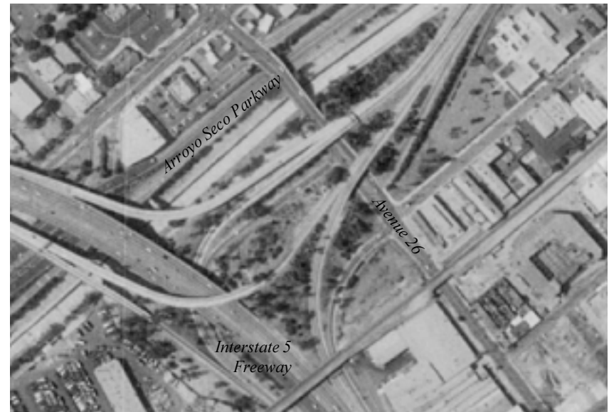
Aerial photo of Avenue 26/Interstate 5 area
