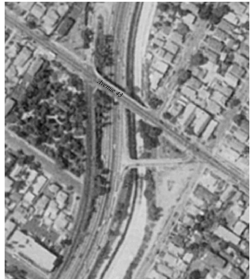
Aerial photo of Avenue 43 offramp
