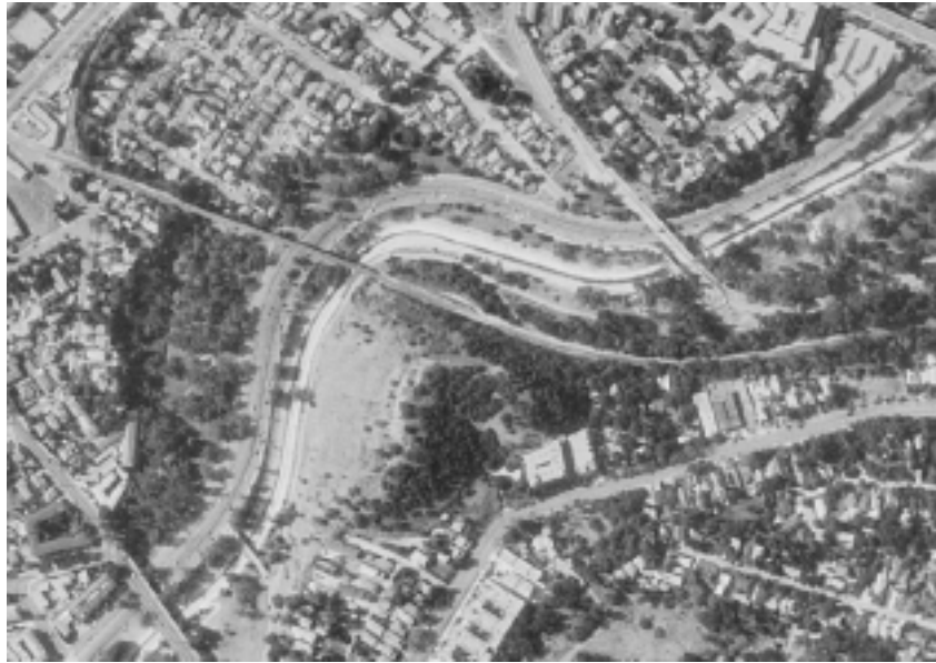
Aerial view of southbound turnout site
