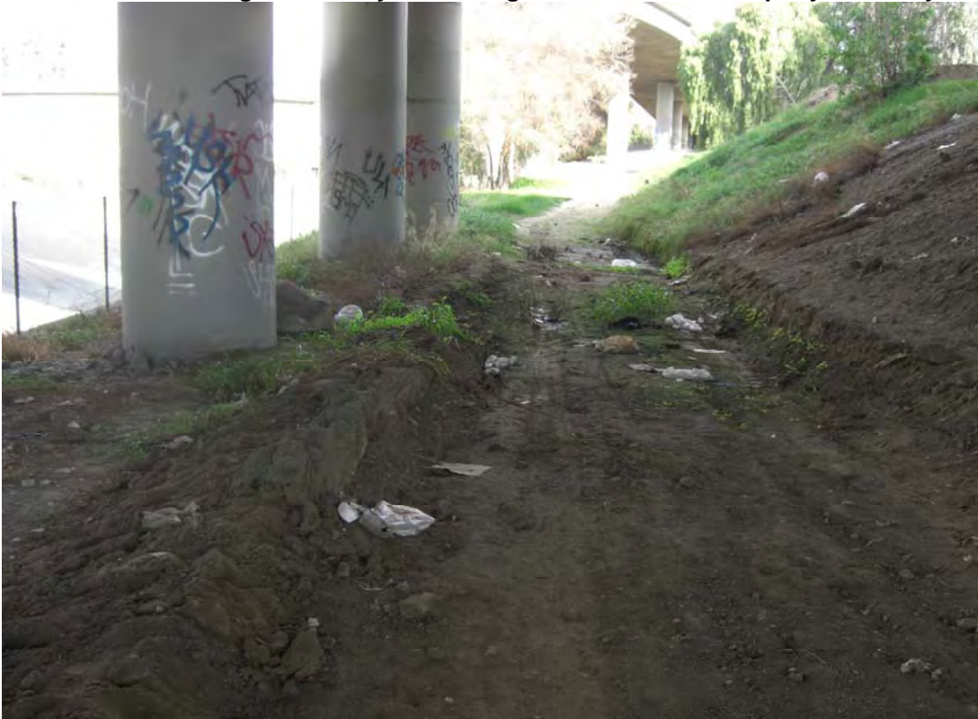
Looking North - Under Interstate 5 ramp
