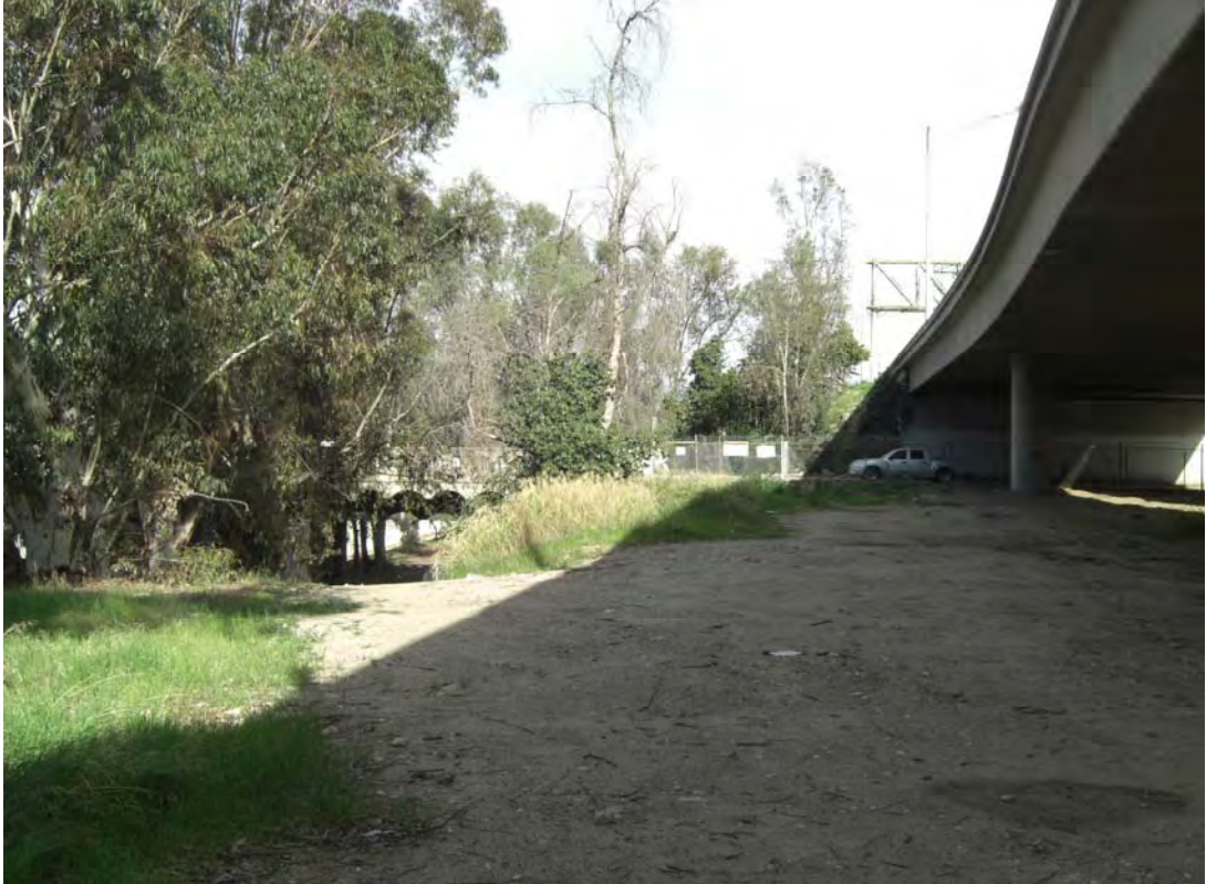
Looking North - Under Freeway Ramp looking at Avenue 26
