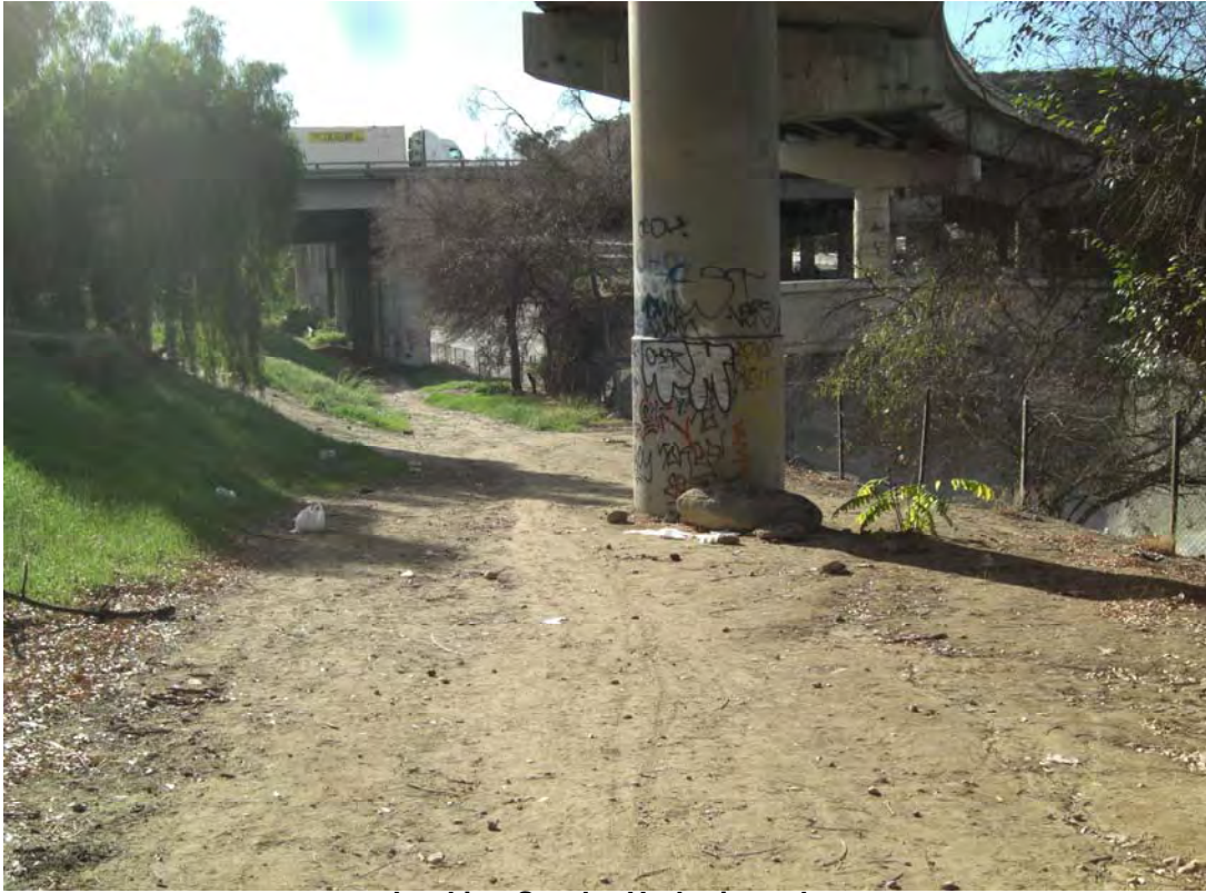
Looking South - Under interchange ramp
