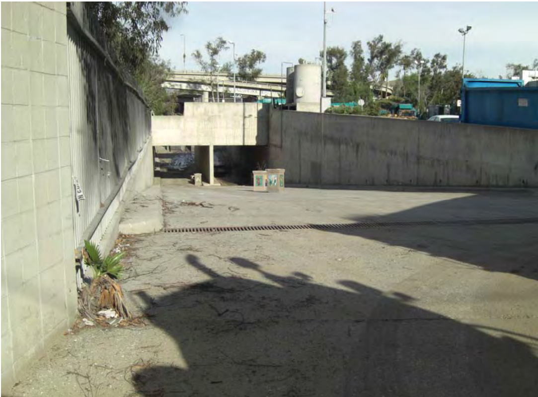
Looking North - Transfer station at City of Los Angeles Sanitation Yard
