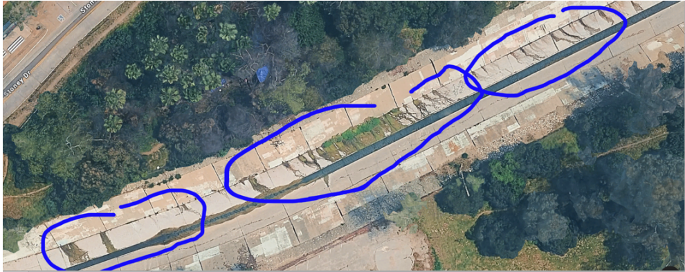
Photo 4 - Visible seepage from San Pascual into channel through eye holes and cracks.
