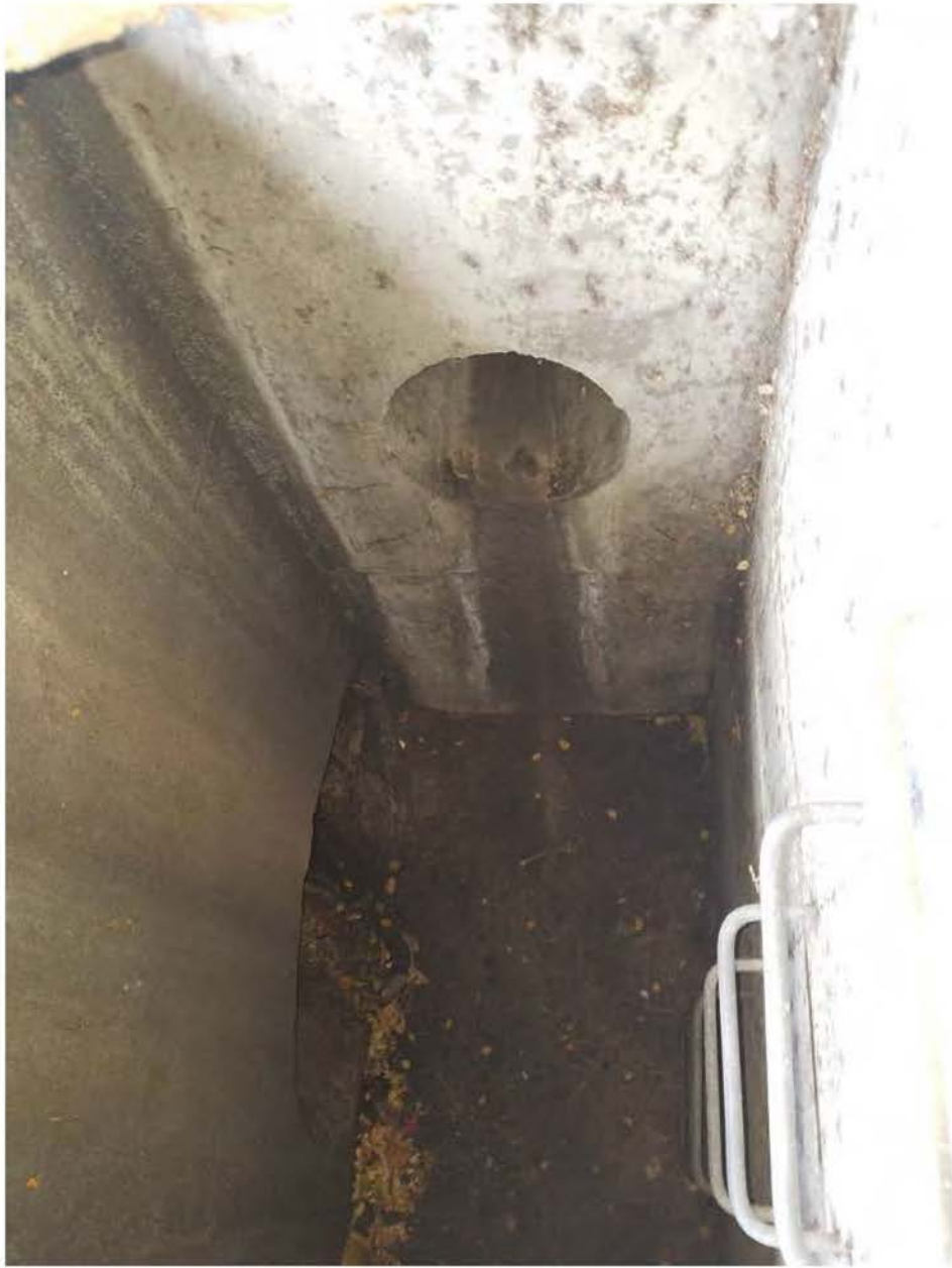
Figure 3. Outfall discharging from the Annandale County Club (Site 1)
