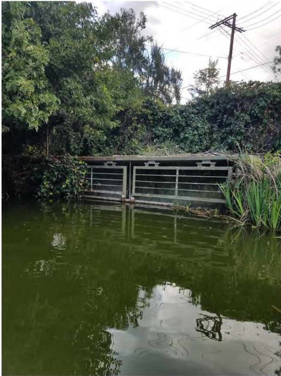
Figure 5. Outfall discharging from lake prior to SD system (Site 3)
