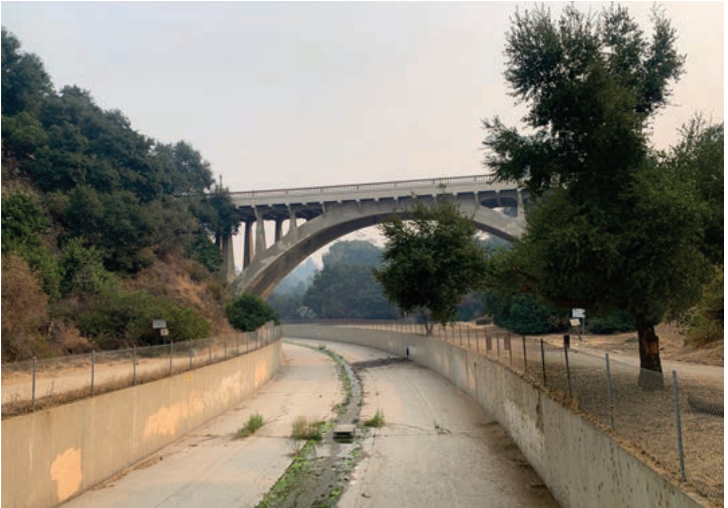
The southern, channelized section of Arroyo Seco beneath San Rafael Bridge. Source: Craftwater Engineering
