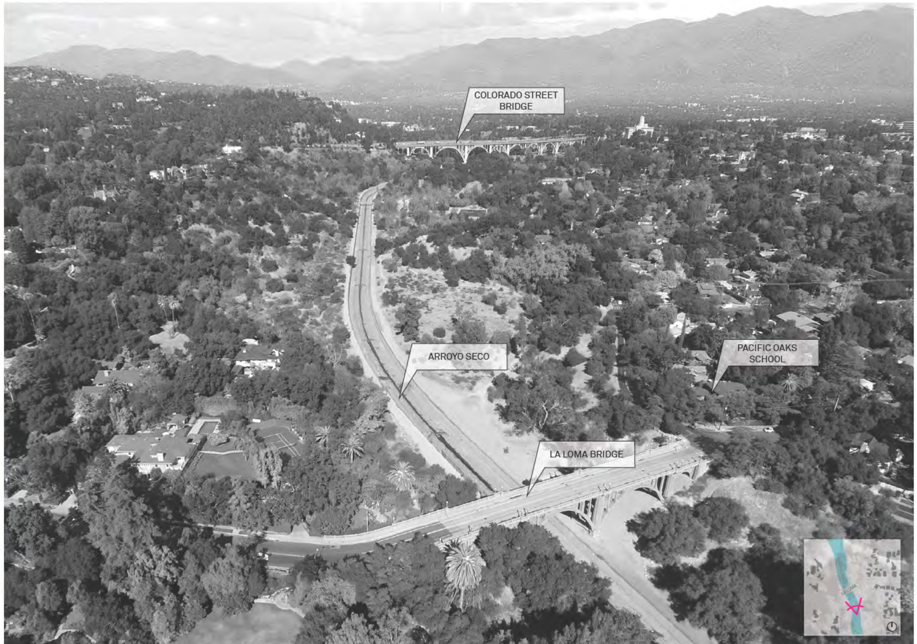
Existing Conditions looking North from Bradford Street
