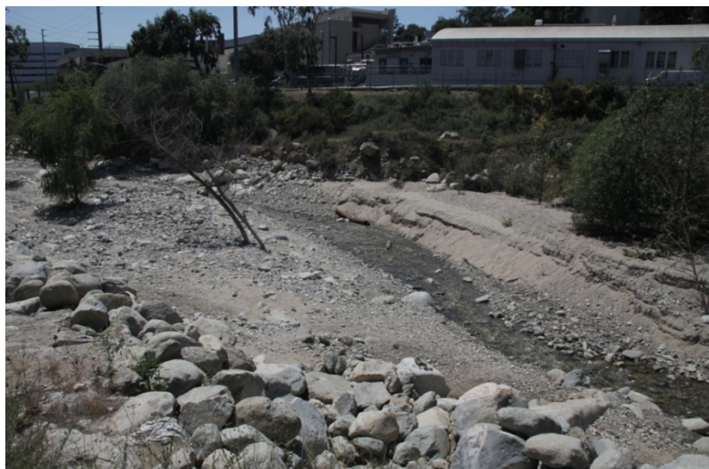
Arroyo Seco Downstream of Los Angeles County Diversion Structure
