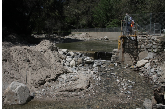
View upstream of Arroyo Seco to Headworks Diversion Structure
