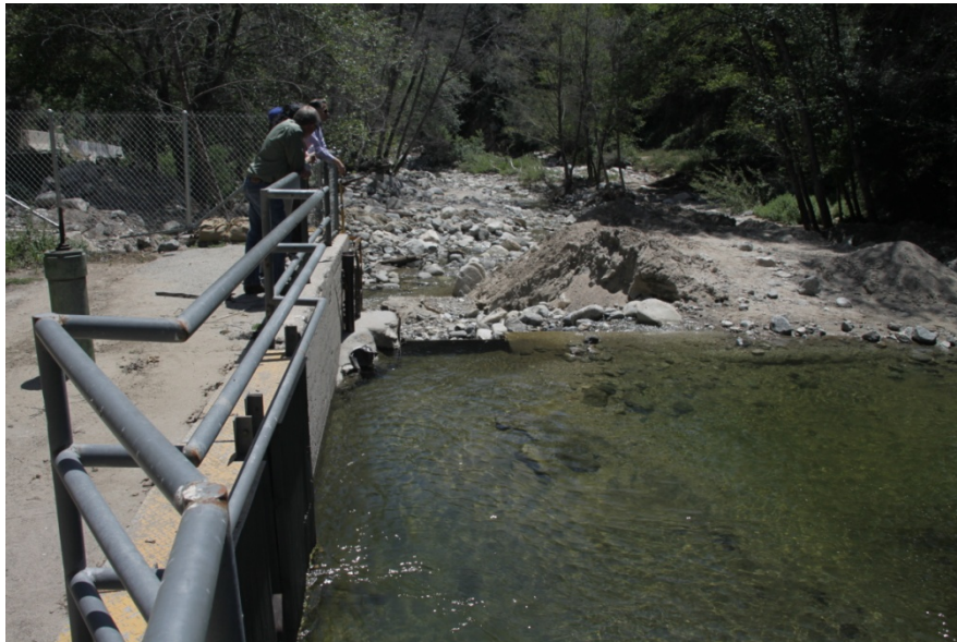
Arroyo Seco Downstream of Headworks Facility
