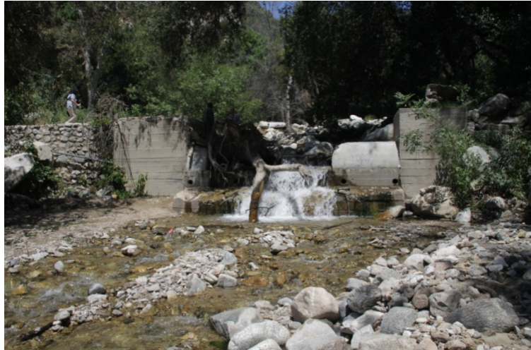
Lincoln Avenue Water Company's Millard Diversion Dam
