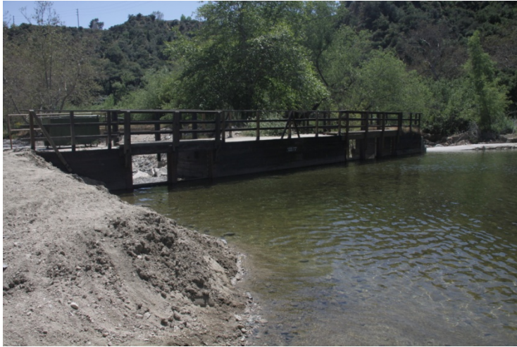
Arroyo Seco at PWP's Headworks Facility
