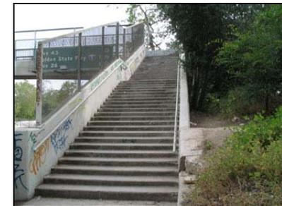
**Figure 52. Stairs on west side of pedestrian bridge restrict bike and wheelchair access**
