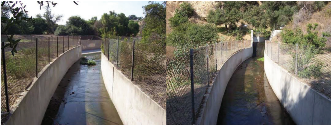
San Rafael Creek channel. Source: Bureau Veritas 2012
