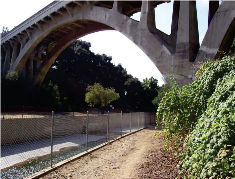
Arroyo Seco Trail at San Rafael Ave Bridge. Source: Bureau Veritas 2012
